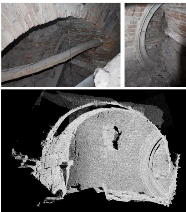
Figure 4. Photos and pointcloud representing the indoor side of the façade wall in the extreme eastern attic. Top left: photo of a big arch in the façade wall, over the chapel rows, in right attic. Top right: Detail of a closed window in the wall under the arch. Bottom: pointcloud view of the same element of top images.
